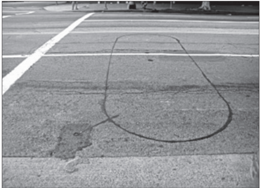
Figure 4. Smart transit priority detector.
