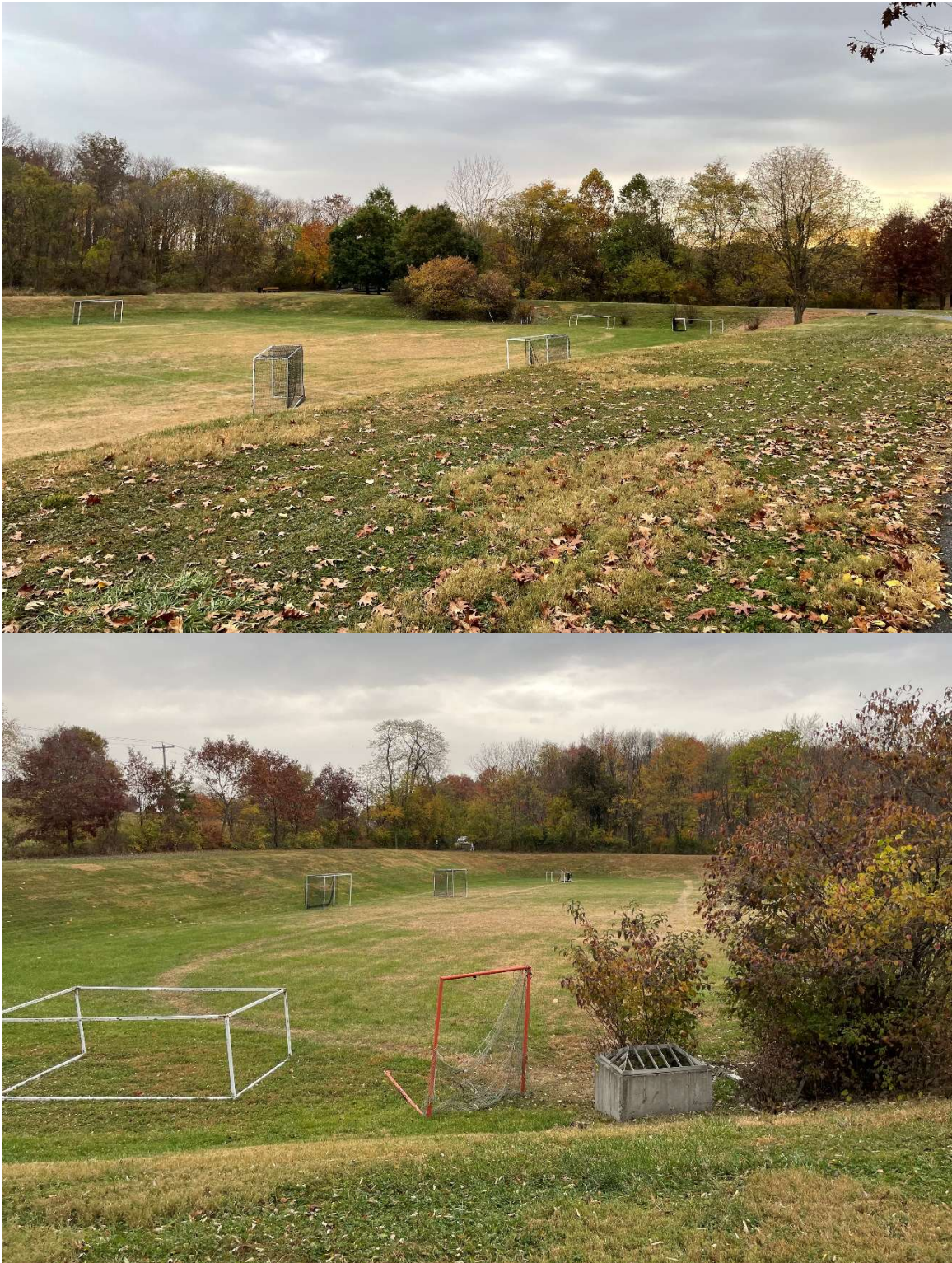
Figure B-7. A floodable recreational space using berms along the perimeter of the field and an inlet structure to control the water level
