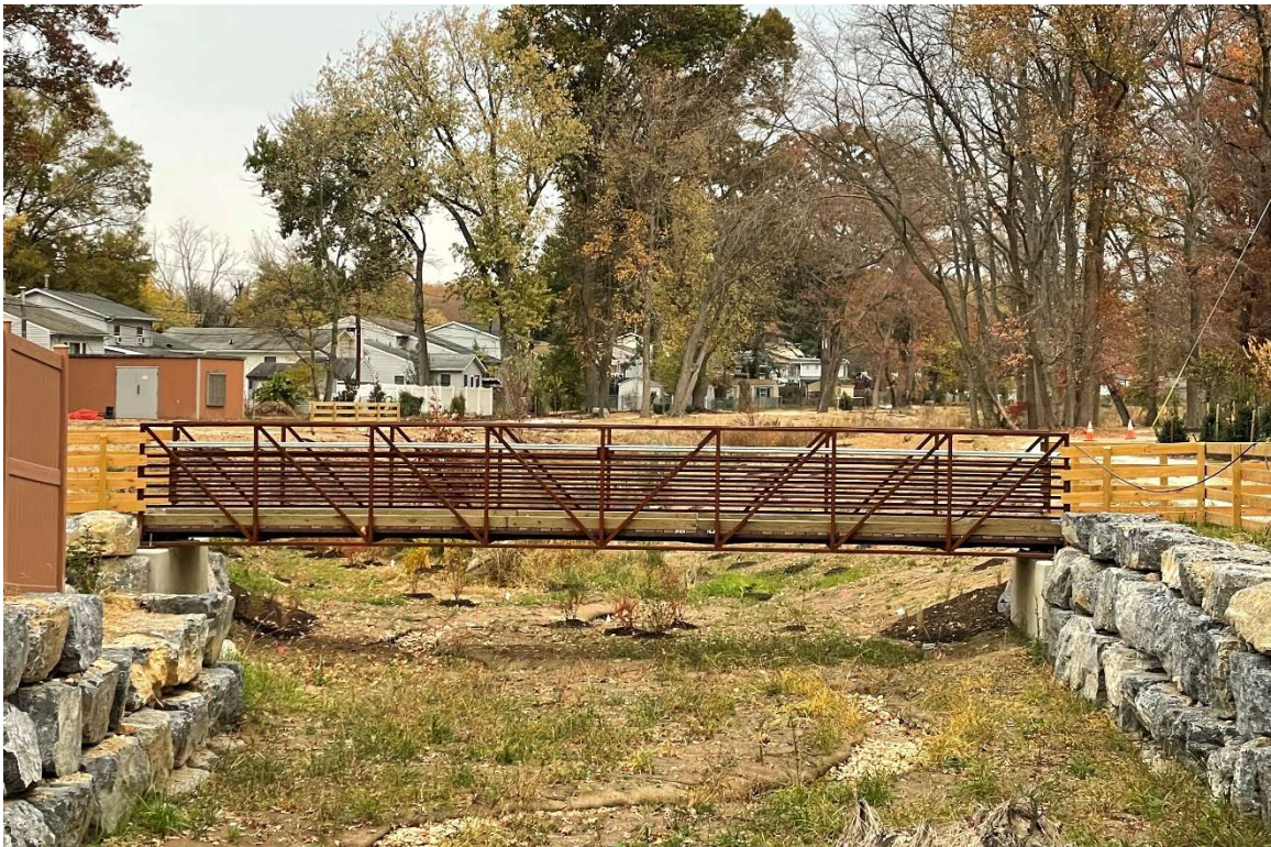
Figure B-2. A completed stream restoration project with a pedestrian crossing using imbricated rock walls to maximize space for floodplain
