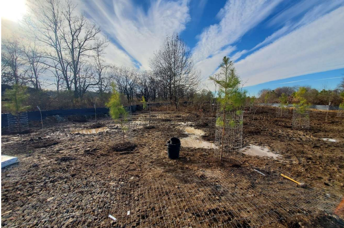
Figure B-12. Tree planting enhanced with soil amendment to maximize storage and infiltration
