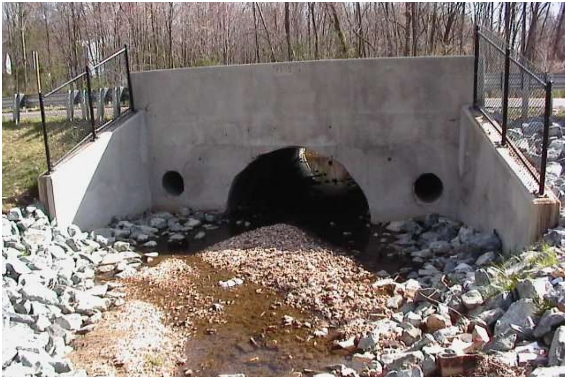
Figure B-16. Completed culvert modification with multiple pipes
