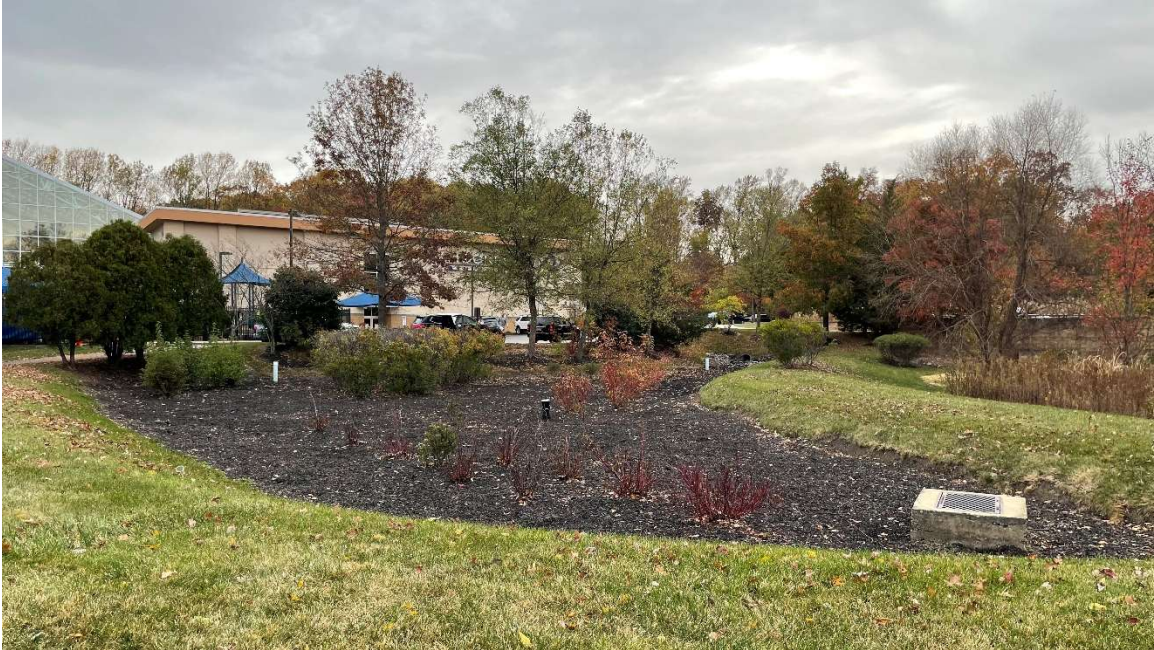
Figure B-9. Completed bioretention area in an urban community
