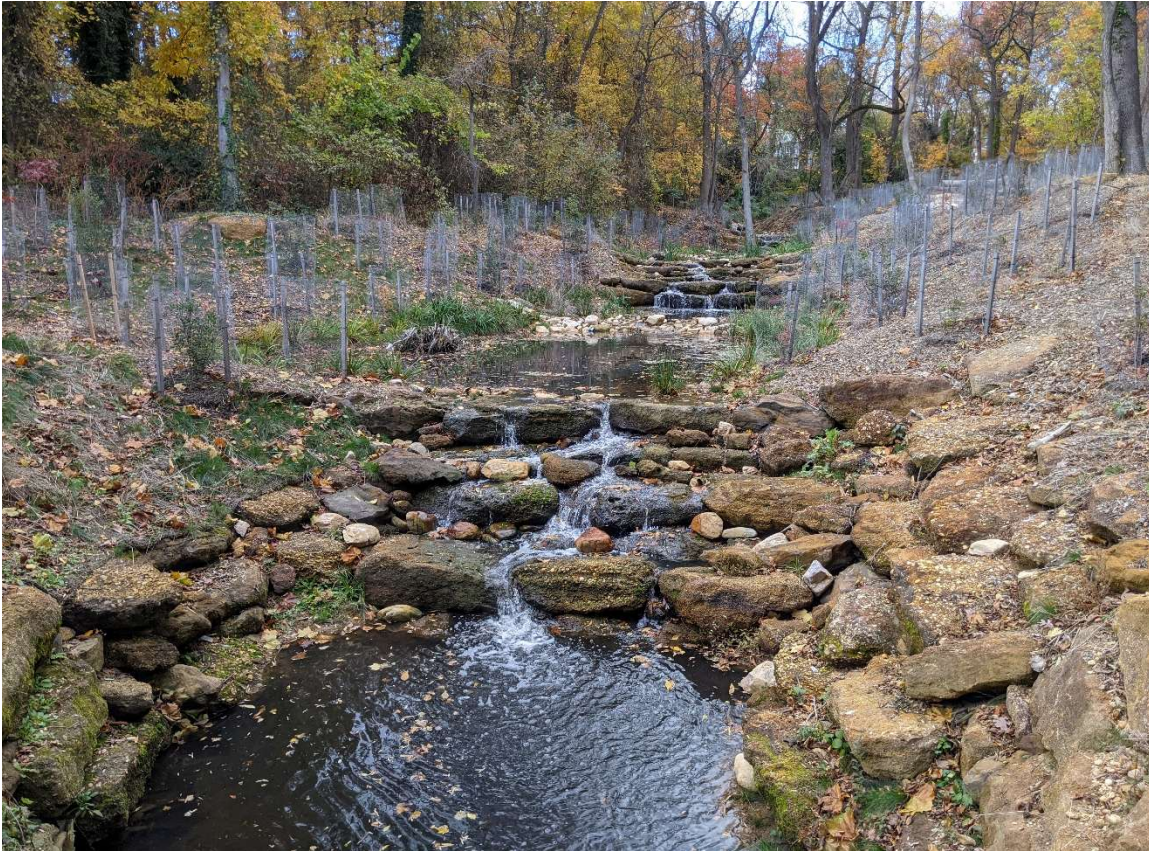
Figure B-17. Completed outfall retrofit using a step pool stormwater conveyance system
