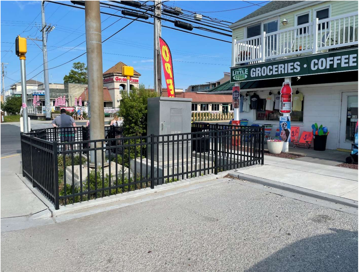
Figure B-6. A completed blue-green street with permeable pavement and bio-retention area
