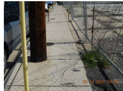
Figure 2-28: Tier 2 Sidewalk Segment
