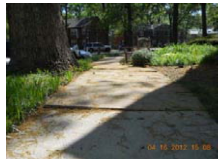
Figure 2-35: Tier 3 Sidewalk Segment
