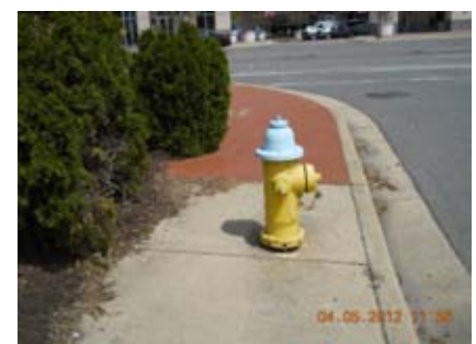
Figure 2-31: Fire Hydrant as Obstruction
