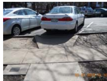
Figure 2-4: Obstructed Curb Ramp
