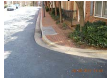
Figure 2-5: Ramp is Obstructed and Below 36 Inches
