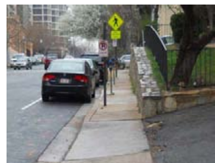
Figure 2-25: Tier 1 Sidewalk Segment
