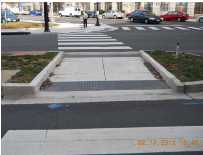
Figure 1-16: Wide Median with Truncated Domes
