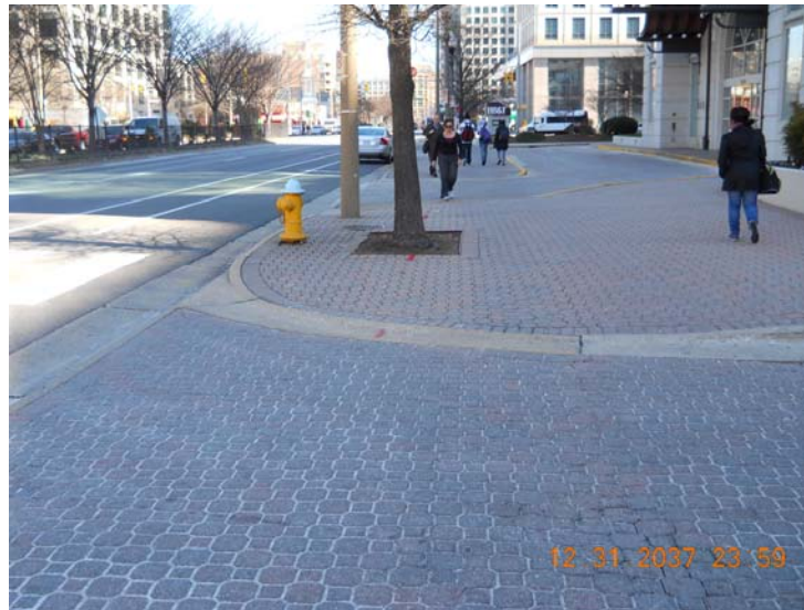
Figure 1-10: Example of Depressed Corner
