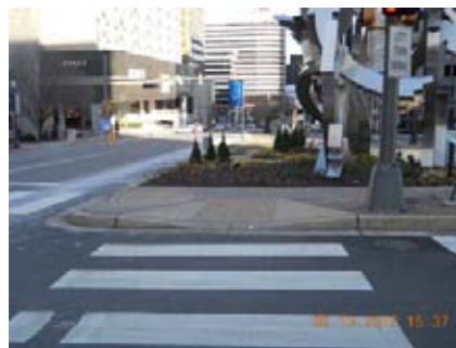
Figure 2-7: Tier 3 Curb Ramp
