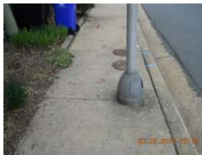
Figure 2-30: Street Light as Obstruction
