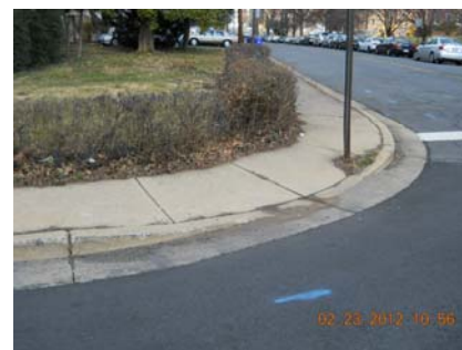
Figure 2-3: Tier 1 Curb Ramp
