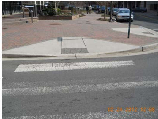
Figure 1-3: Perpendicular Curb Ramps in Arlington, VA
