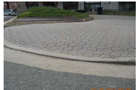
Figure 2-56: Tier 3 Intersection with a vertical change
