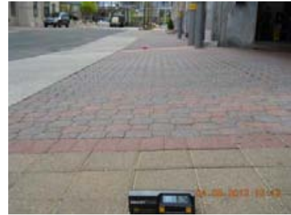
Figure 2-36: Tier 4 Sidewalk Segment
