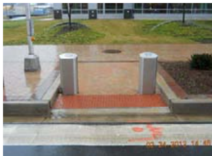
Figure 2-8: Tier 4 Curb Ramp
