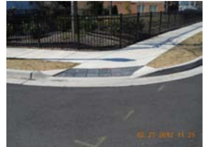
Figure 2-9: Non-Functional Flares
