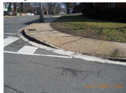
Figure 2-6: Tier 2 Curb Ramp
