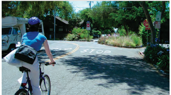
An example from Berkeley of a diagonal diverter in a residential neighborhood | Source: NACTO
