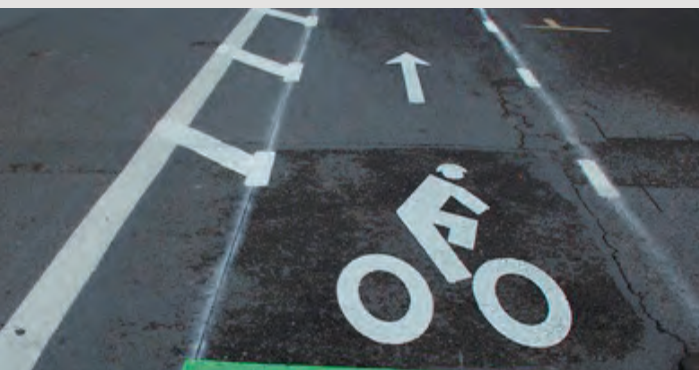
A bike lane with a paint buffer to provide some distance between motor vehicles and bikes | Source: KAI
