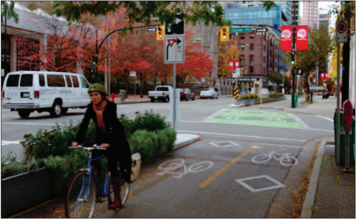
Separated Bike Facility in Vancouver, BC; Source: Paul Krueger
