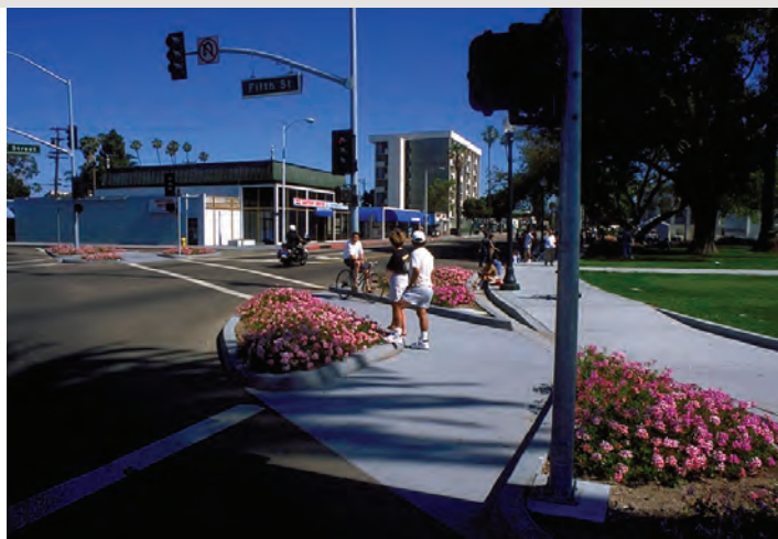
Curb Extensions in Oxnard, CA; Source: Dan Burden
