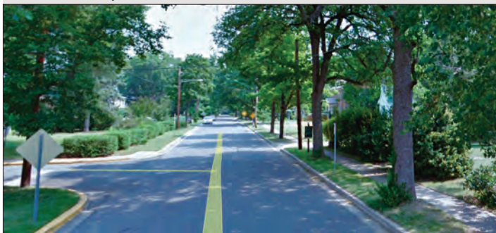
Dartmouth Avenue - College Park, MD; Source: Google Streetview, 2015
