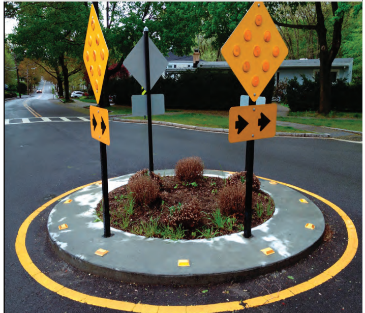
Mini roundabouts slow cars using horizontal deflection. This is the same strategy employed by chicanes and checkered parking patterns : NACTO
