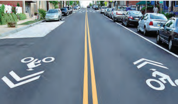
Sharrows; lowest separation bicycle facility | Source: KAI
