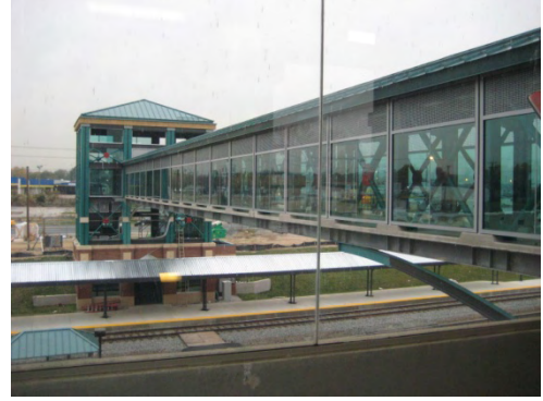
Figure 24: Pedestrian Overpass, Woodbridge, VA (VRE)
