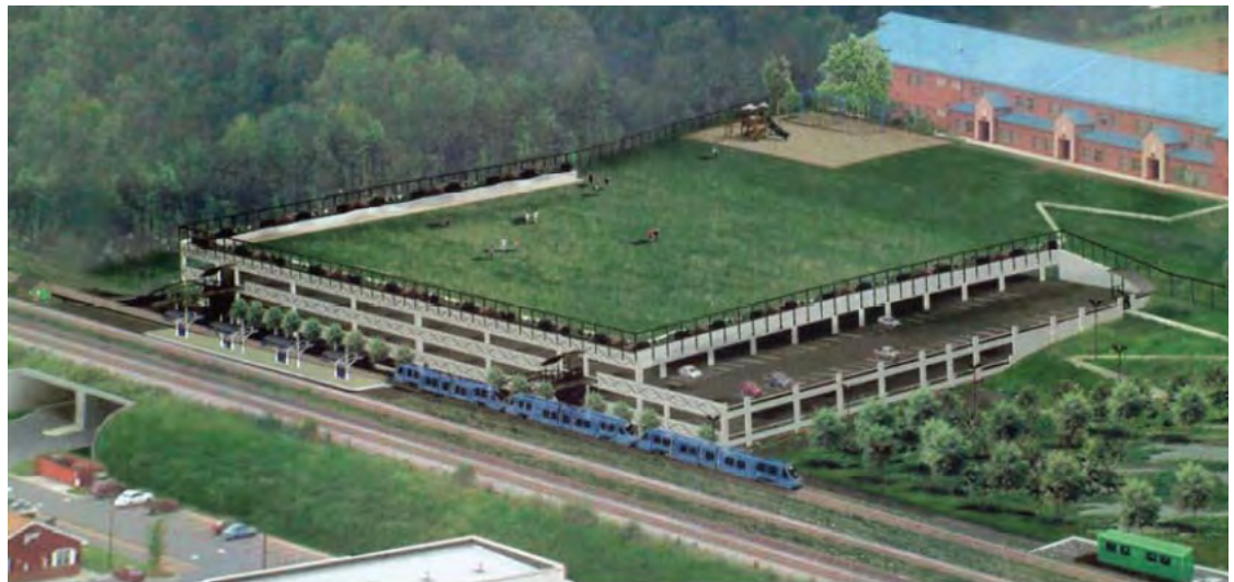
Rendering of the I-485/South Boulevard Station, showing Sterling Elementary School and playground on the garage rooftop.
