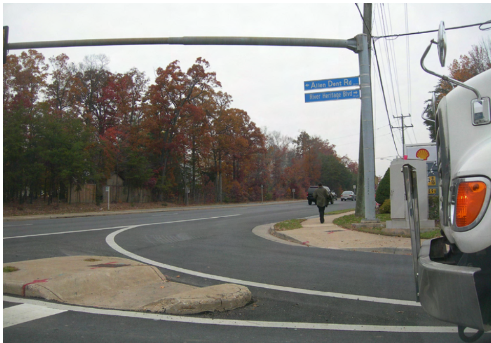
Figure 6: Missing Crosswalks, Auto-Oriented Land Use on River Heritage Blvd
