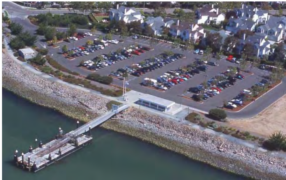
Figure 7: Bay Farm Ferry Terminal
