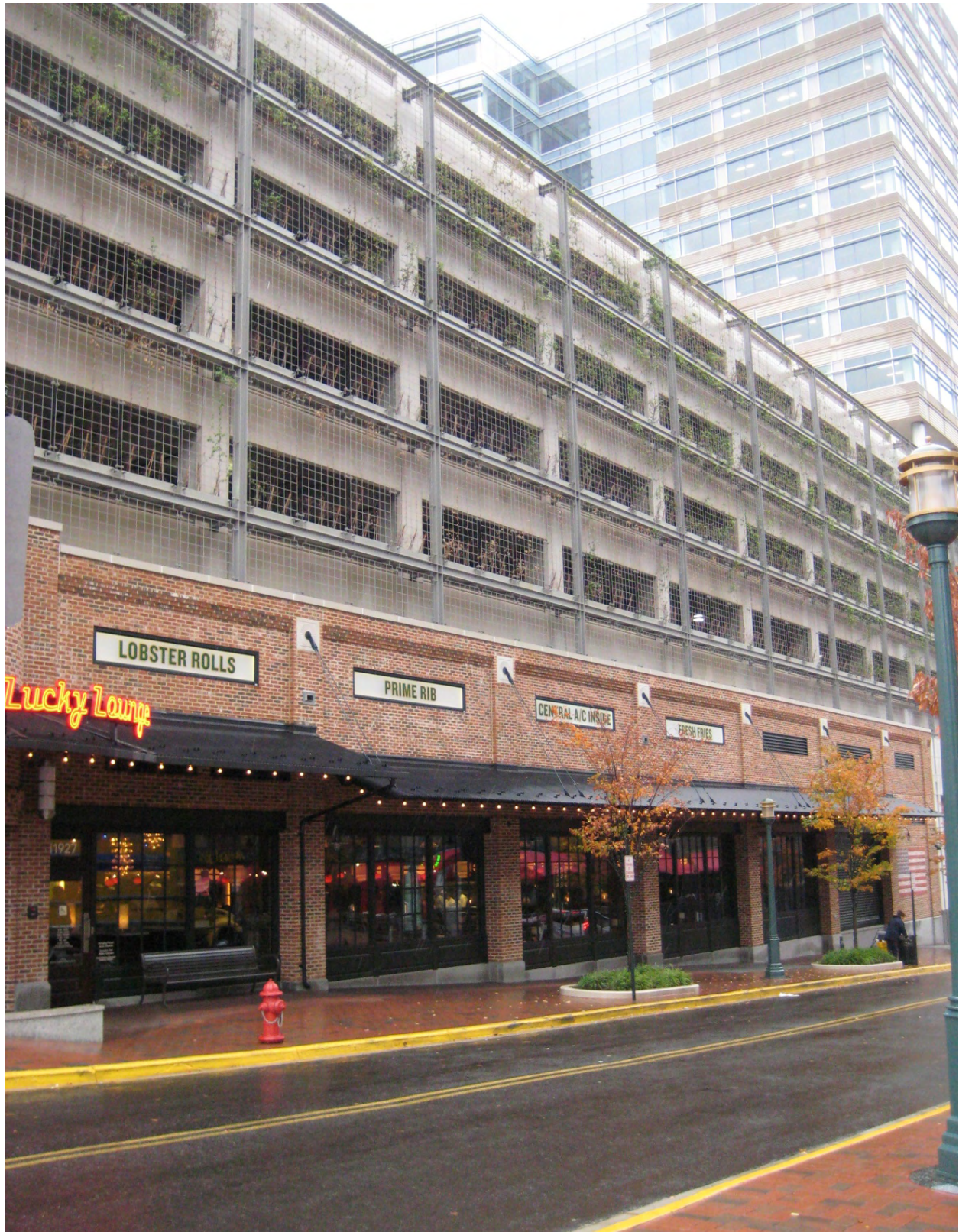
Unique architecture, parking with ground floor retail to preserve pedestrian experience at street level, pedestrian scale lighting, wide, tree-lined sidewalks
