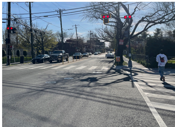
DDOT recently upgraded a rectangular rapid flashing beacon (RRFB) to a HAWK signal on Alabama Avenue SE to better control traffic.
