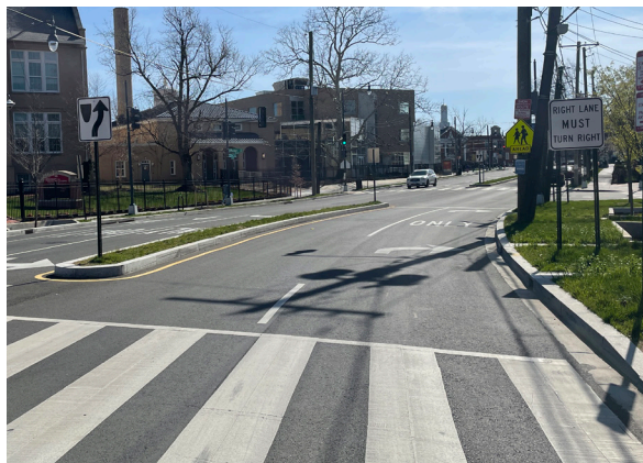
DDOT installed new medians, crosswalks, and landscaping along Martin Luther King Jr. Avenue SE in 2021.
