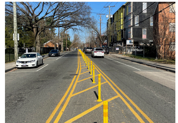
As part of the Alabama Avenue SE safety improvements, DDOT added median flexposts to calm traffic and restrict turning movements in certain locations.
