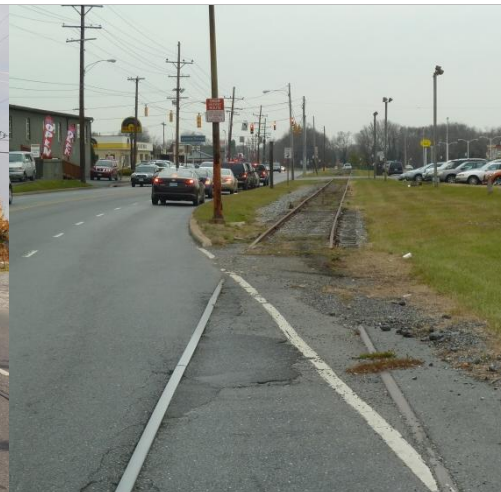
FIGURE 3-4: RAIL TRANSITION LOCATION, NORTH OF E. 8 TH ST., LOOKING NORTH
