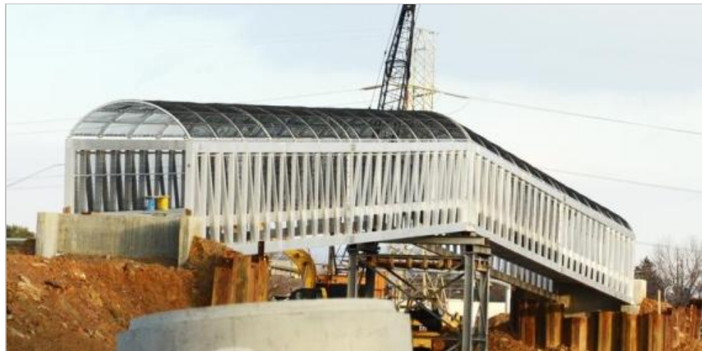
FIGURE 3-22: MOTTER AVE TEMPORARY BRIDGE
