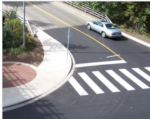
FIGURE 2-8: HIGH VISIBILITY MARKINGS
