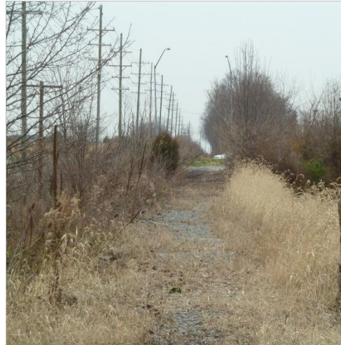
FIGURE 3-5: INACTIVE RAIL, SOUTH OF LIBERTY ROAD, LOOKING NORTH
