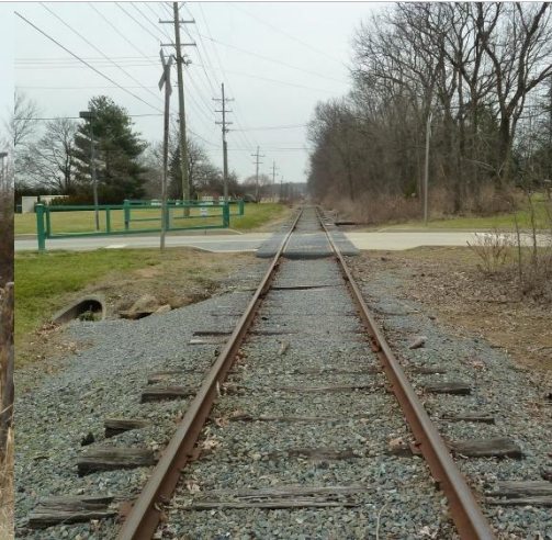
FIGURE 3-6: ACTIVE RAIL, NORTH OF LIBERTY ROAD, LOOKING NORTH
