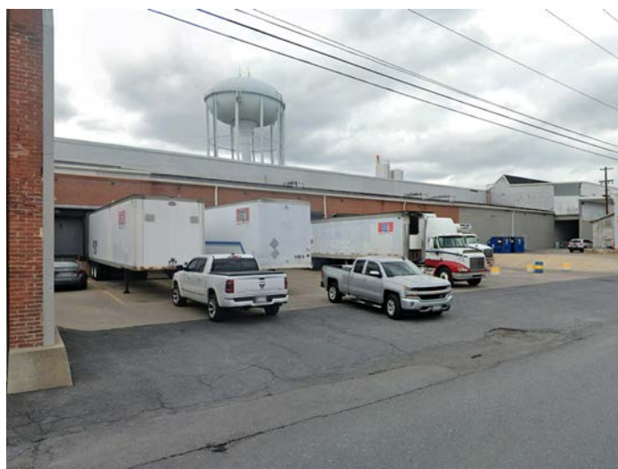
No sidewalks are present at the Dairy Maid location between 7th and 8th Street. Pedestrian safety and comfort are further jeopardized by the circulation pattern of large trucks backing into the loading dock.
