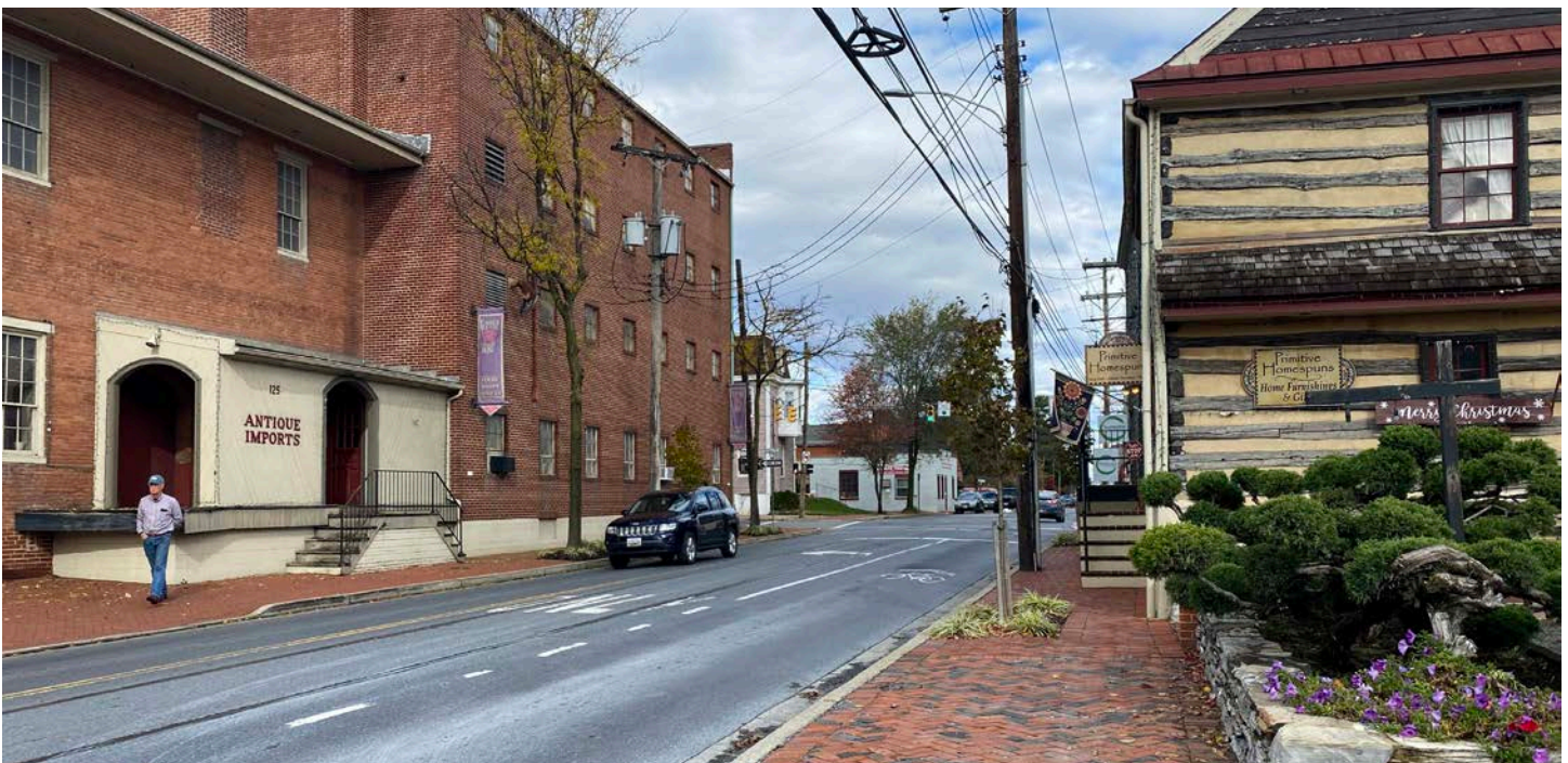
View of the historic downtown area segment of East Street looking north towards the 2nd Street intersection.
