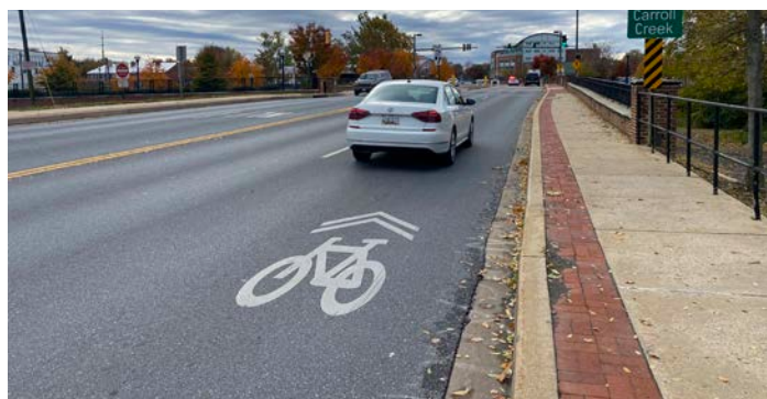
Existing sharrows on East Street between the MARC station and 7th Street.
