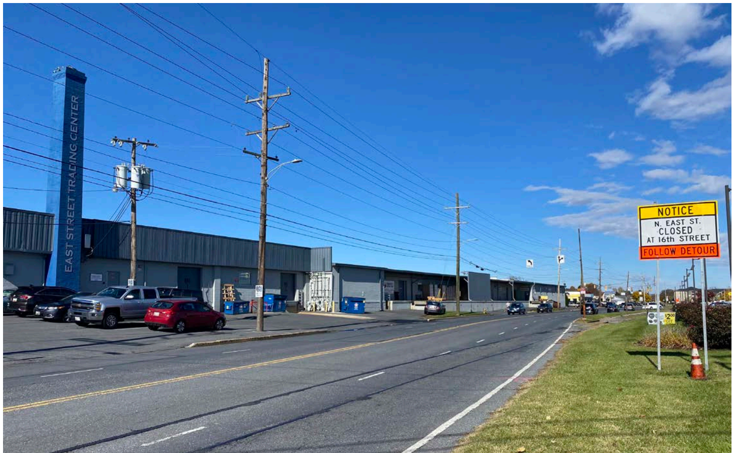
View of East Street looking north towards 5th Street. This segment lack sidewalks on both sides of the street. A spur of the abandoned rail tracks crosses the 'Sharrow' or shared outside travel lane and is a safety concern for people on bicycles.
