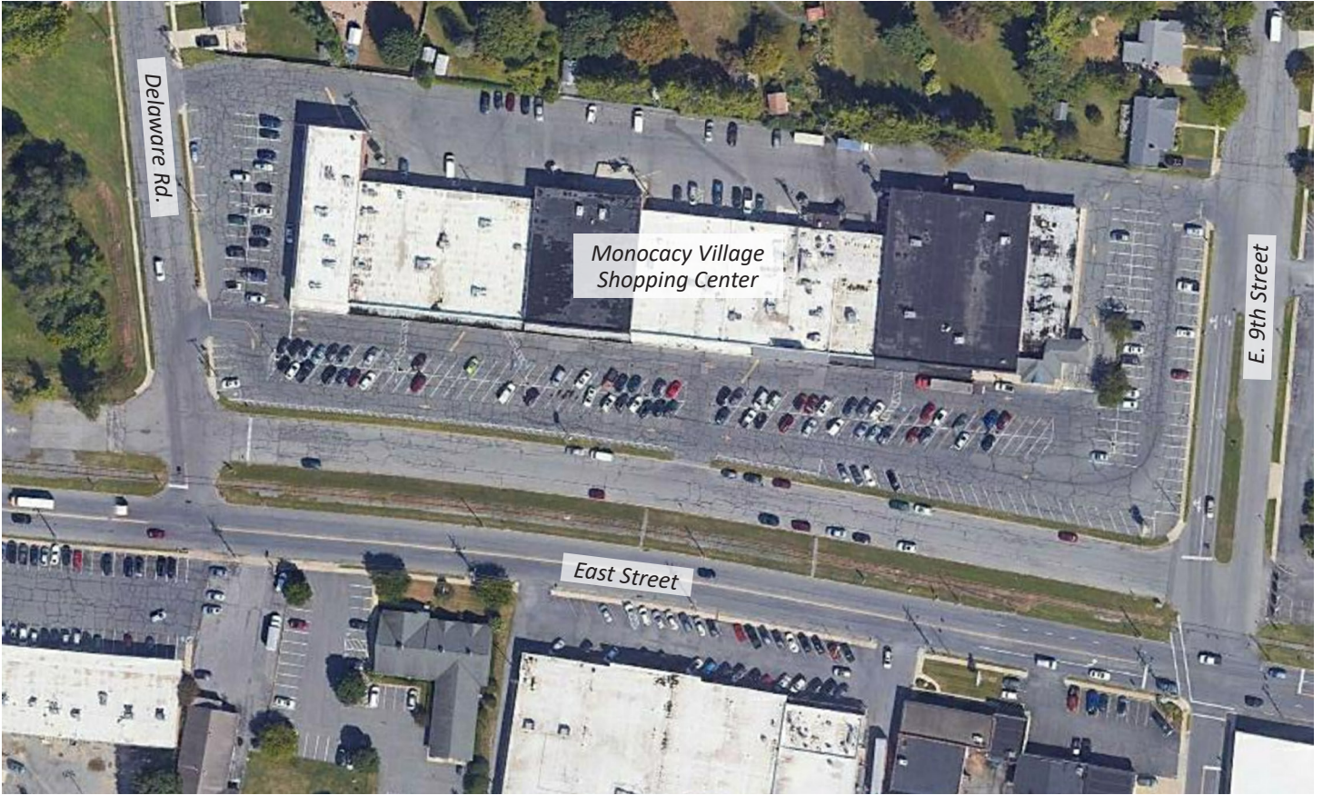
Figure 5.39: Monocacy Village Shopping Center (existing conditions)
