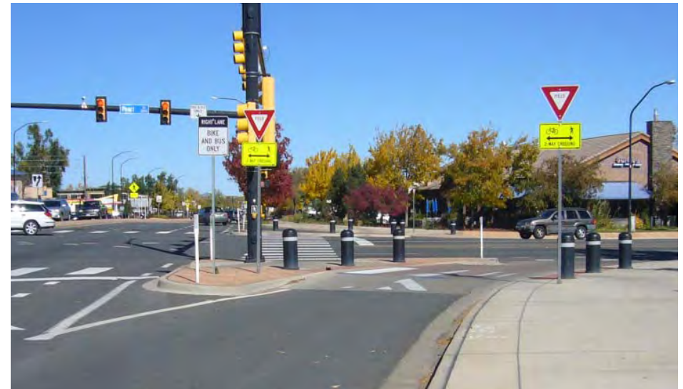
FIGURE 15 | EXAMPLE OF A RAISED CROSSWALK IN BOULDER, CO
