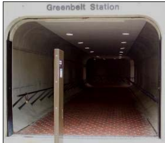
Figure 4-5: Tunnel access from the west side of the Greenbelt Metrorail station.
