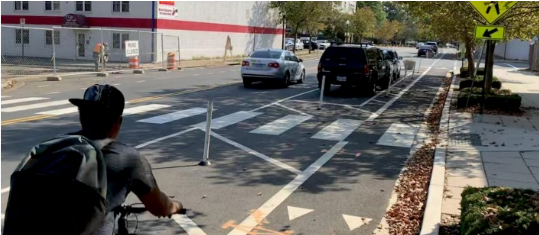
Figure 30. Roadway elements adjacent to the curb including parking protected bike lanes are currently not included in the curb space allocation tool
