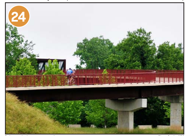
Pedestrian bridge connection at Anacostia.
