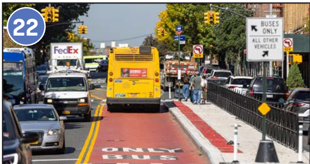
Dedicated bus lane separating transit users from passenger vehicles
