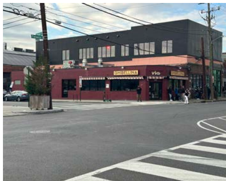
Missing crosswalk on Fenwick Street
