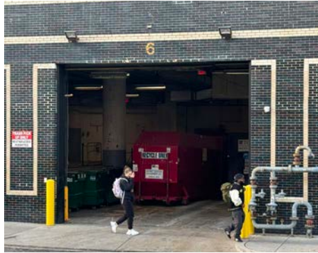
Open service garages
