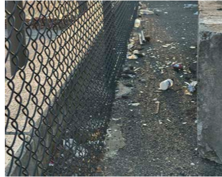
Excessive litter and broken glass
