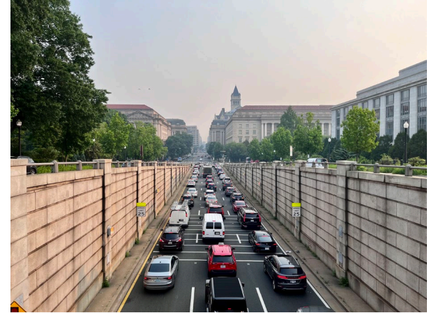
Traffic congestion on 12 street tunnel, downtown DC (Joe Flood/Flickr)
