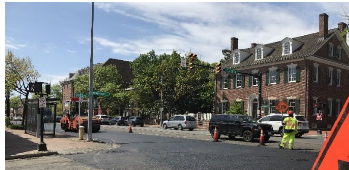
Street repaving in Alexandria, VA (Rachel Beyerle/COG)
