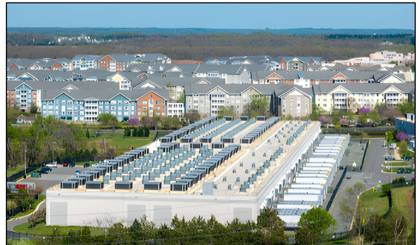
Amazon data center, Loudoun County (source: VCNVA )
