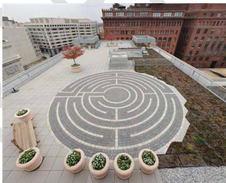
WRI green roof (Source: www.apabuilding.com )
