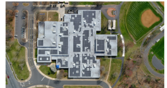
Beville Middle School solar array
