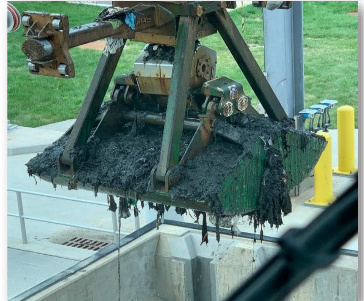
Trash, Debris and Solids Removal from Screening Shaft at Tunnel Dewatering Pumping Station
