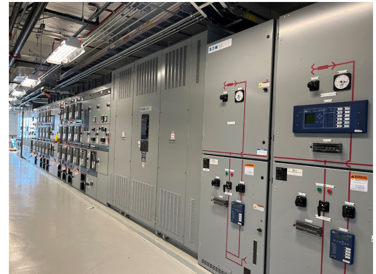
Fig. 3 (TOP): Depot Substation West Elevation. Fig. 4 (BELOW): Depot Substation 13.2Kv Switchgear
