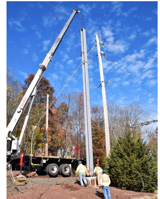
Fig. 2. New steel catenary polls installed along Gladstone ROW.
