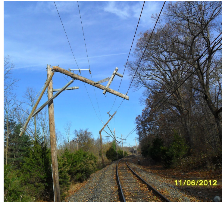
Fig. 1. Damage from Superstorm Sandy to catenary polls along Gladstone Branch commuter line.
