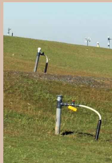
Landfill gas recovery (methane) system in Fairfax County at the landfill
