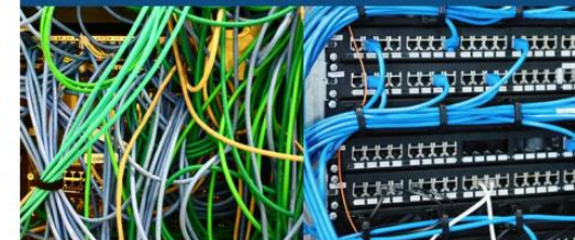
Above: (Left) Example of bad cabling in a data center, (Right) an example of good cabling.
