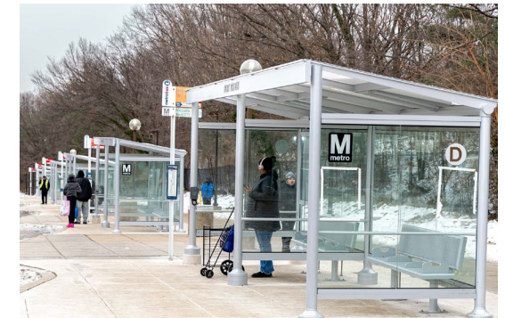
Bus bay assignments & detour signage
