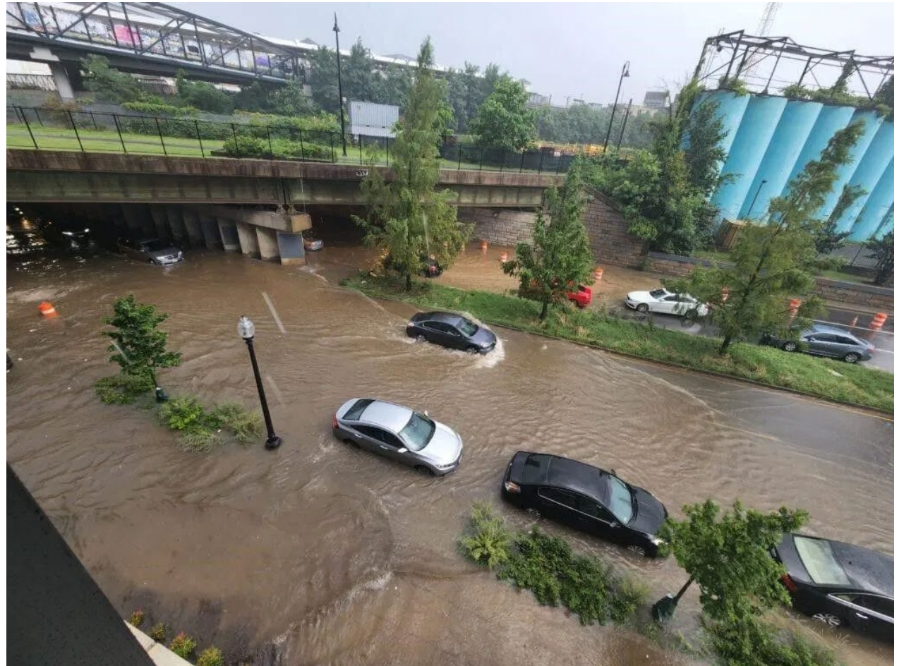
Rhode Island Ave Flooding, 2022 (WJLA)
