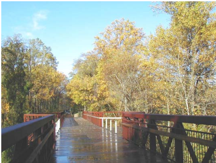
The Capital Crescent Trail Bridge over Rock Creek, Chevy Chase, MD opened in 2003
