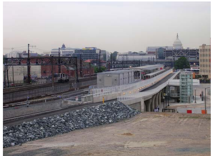
The New York Avenue Metro Station Incorporates a Shared- Use Path and Bicycle Parking
