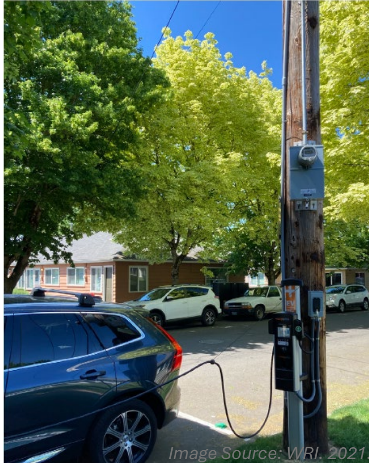
Eye-level pole-mounted charger on utility pole in Portland, OR
