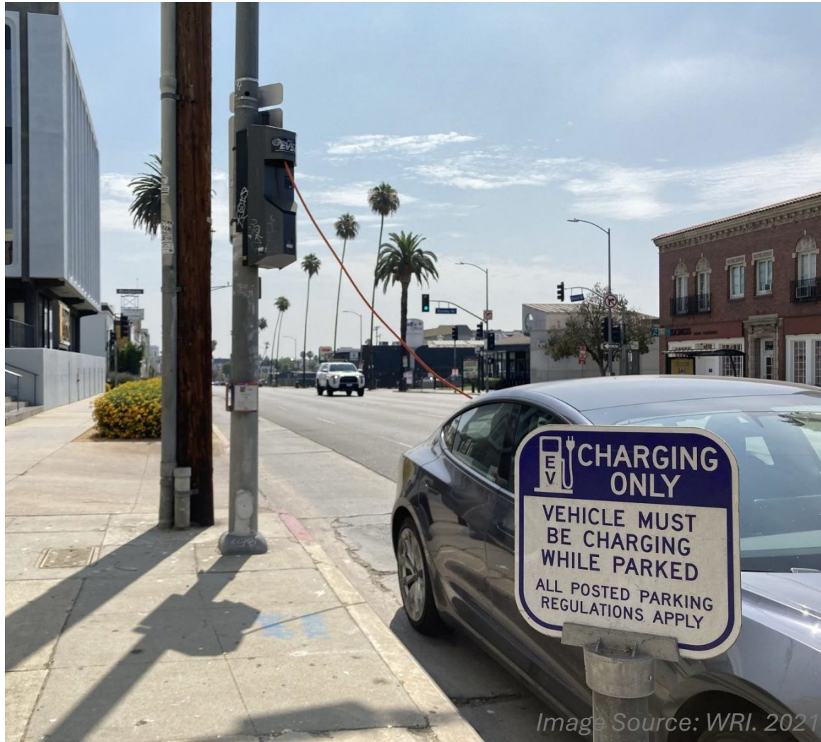
Pole-mounted EV charger in Los Angeles, CA
