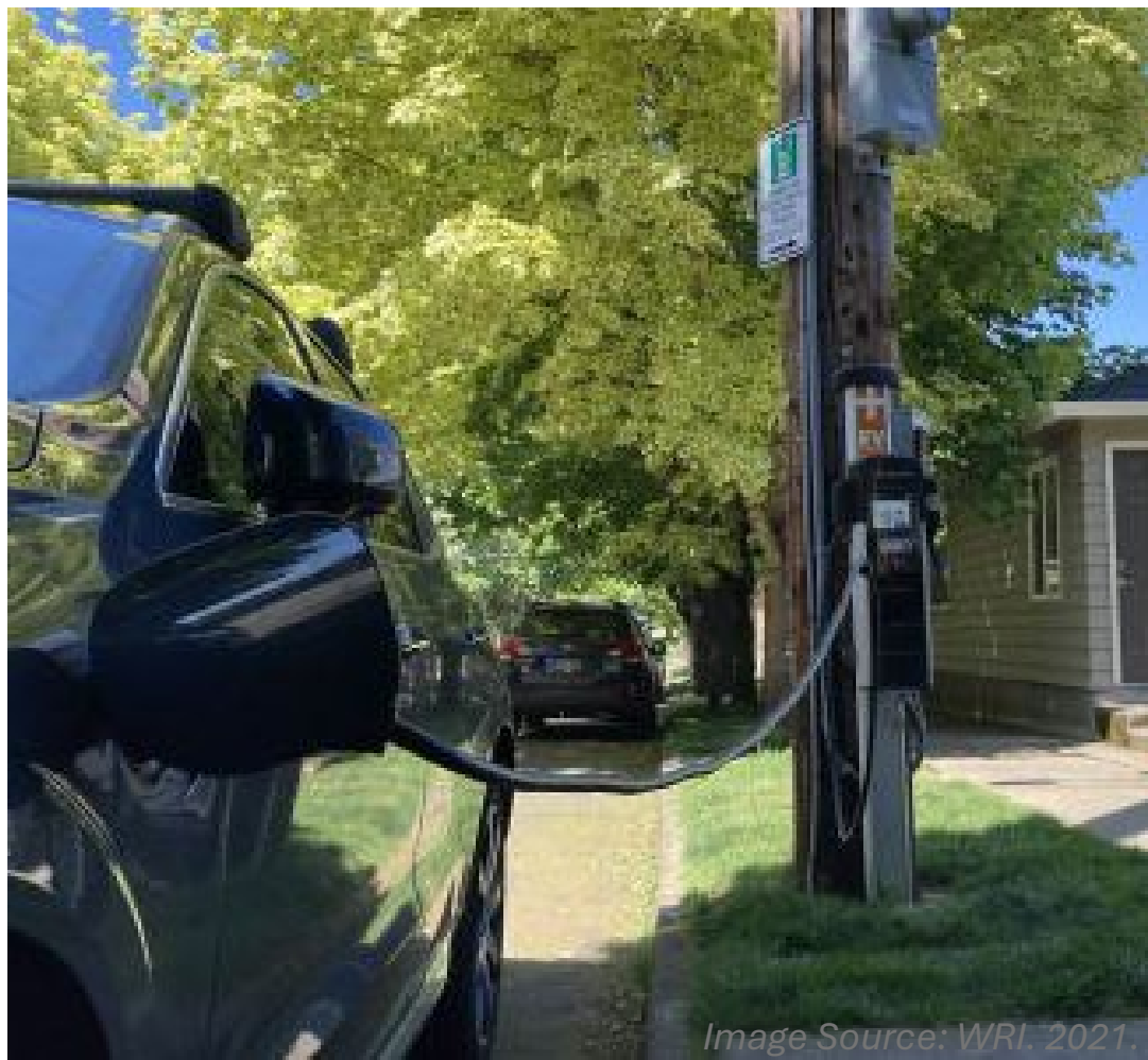
Pole-mounted EV charger in Portland, OR
