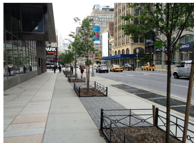
Figure 10. Permeable Paver Step-out Areas. Source: MNLA.
