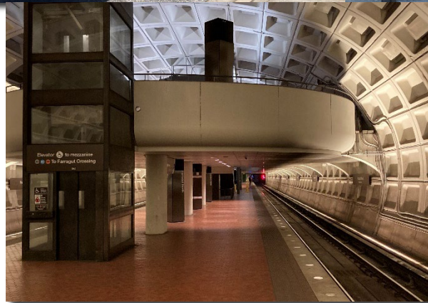
Platform and mezzanine levels of the Farragut North Metrorail station. (Pierre Gaunaurd/TPB)
