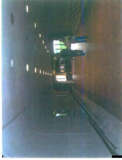
Existing Pedestrian Tunnel Looking @ Station Entrance Mezzanine
