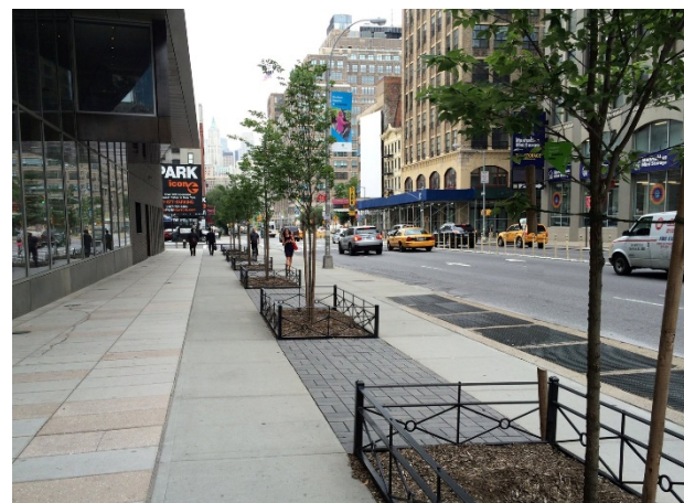
Figure 23. Permeable Paver Step-out Areas. Source: MNLA.
