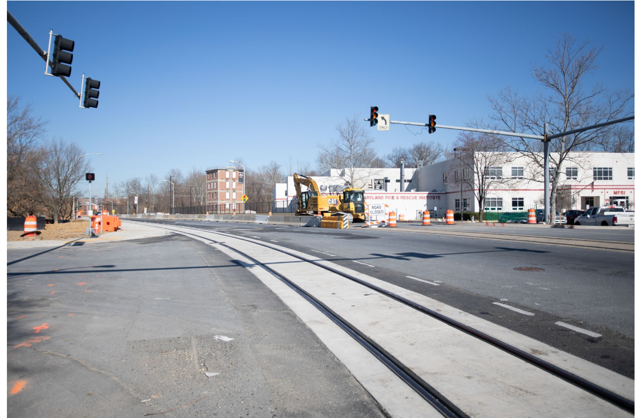
Paving and track installation on Campus Drive near Greenbelt Metro. (Mar. 2025)
