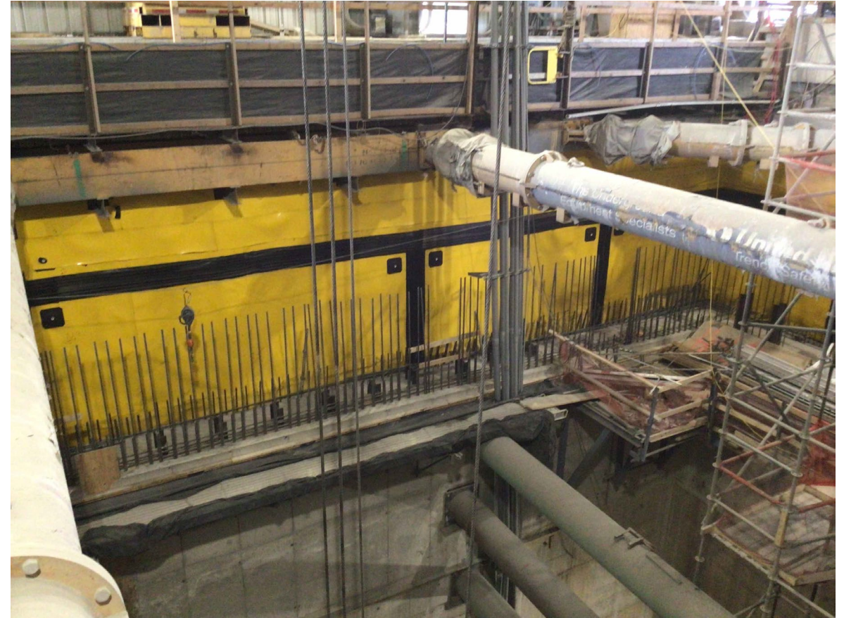
Bethesda Shaft Waterproofing Installation (Mar. 2025)
